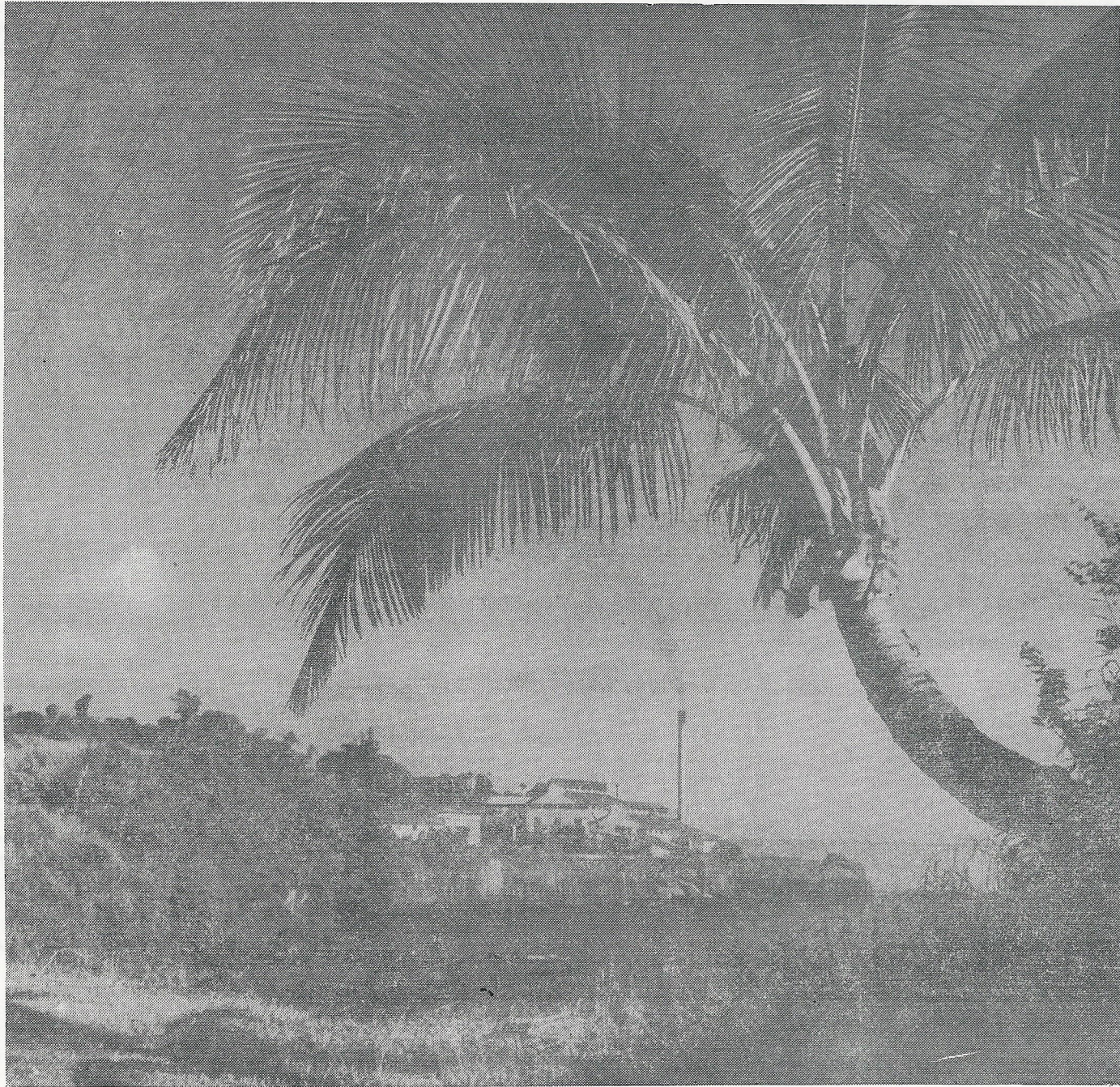
THE FACTORY AT HILO SUGAR COMPANY is shown standing on the shoreline of Hilo Bay. The millyard crane is seen at the left of the line of buildings feeding the cleaning plant. The mill is capable of crushing about 65 tons of cane per hour to produce approximately 780 tons 96 degree sugar per week. In 1957, a new turbine replaced the No. 4 mill at a cost of $50,000. In 1958, replacements were made of six new low grade centrifugal machines, six mill rollers and a boiler was improved at a cost of $135,000, $12,000, and $20,000 respectively.
